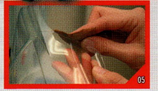
Now smooth the cut edges with sand paper (e.g. 150). Be careful not to loosen the protection film!
